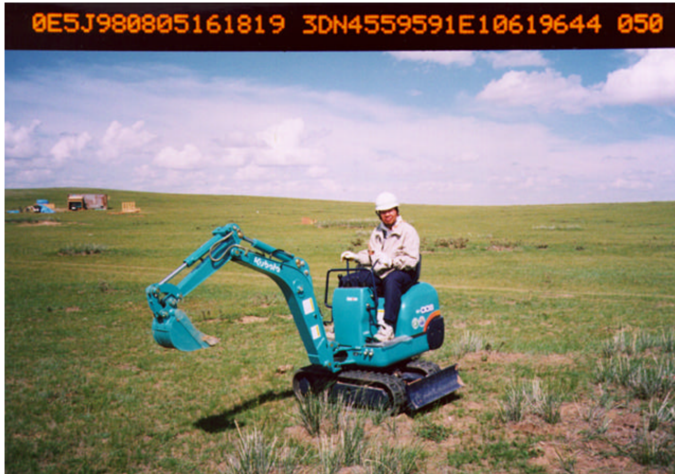
Power Shovel for Making Trench
